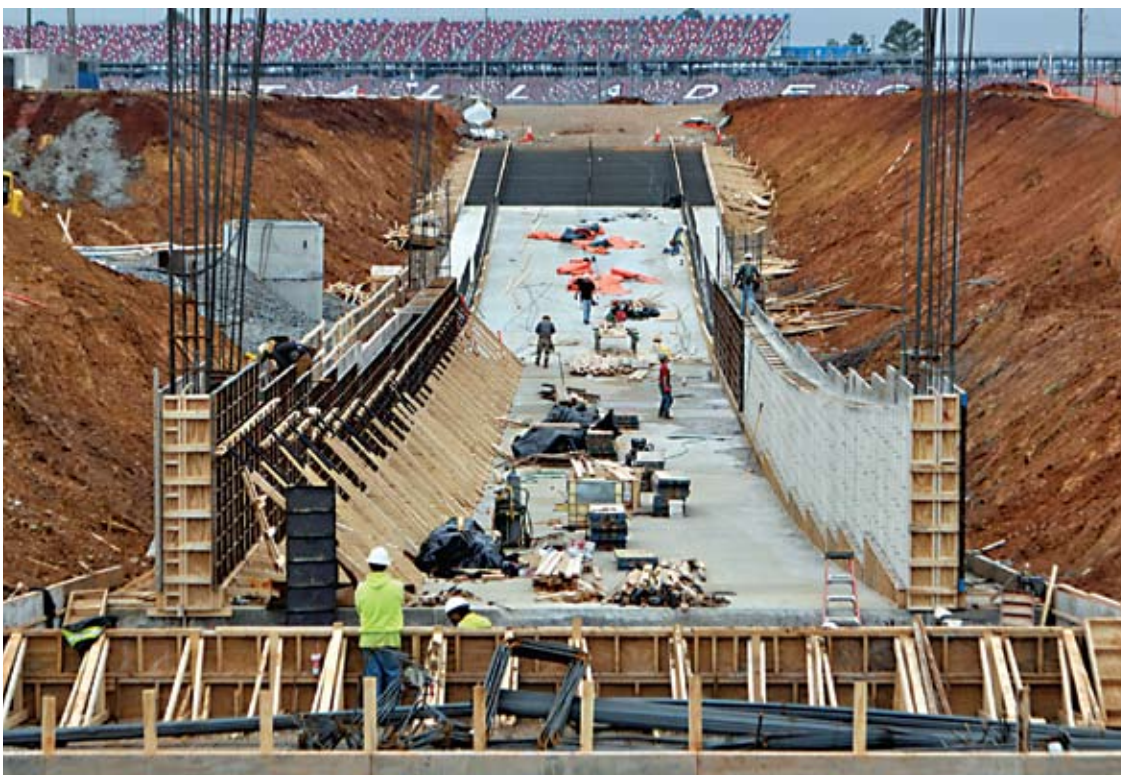
January 2019 progress on the new tunnel at Talladega
