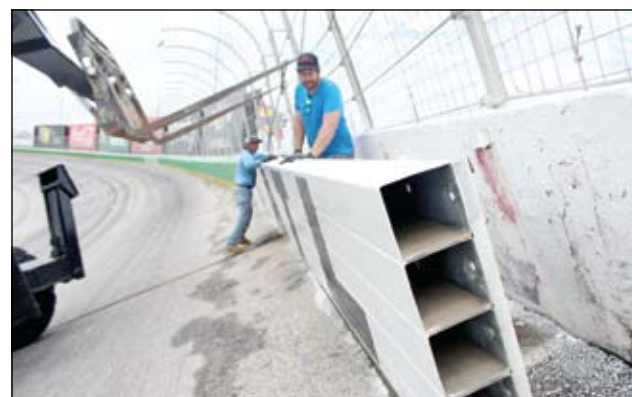
AFTER RACE SAFETY WALLS COME DOWN FOR TRACK RECONSTRUCTION
