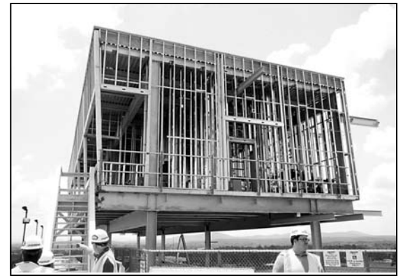
NEW PRESS BOX GOING UP
