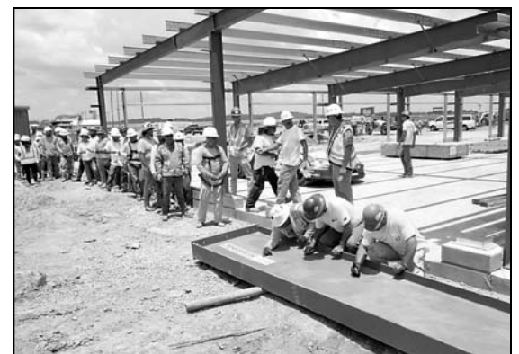
SIGNING OF FINAL MAIN BEAM
