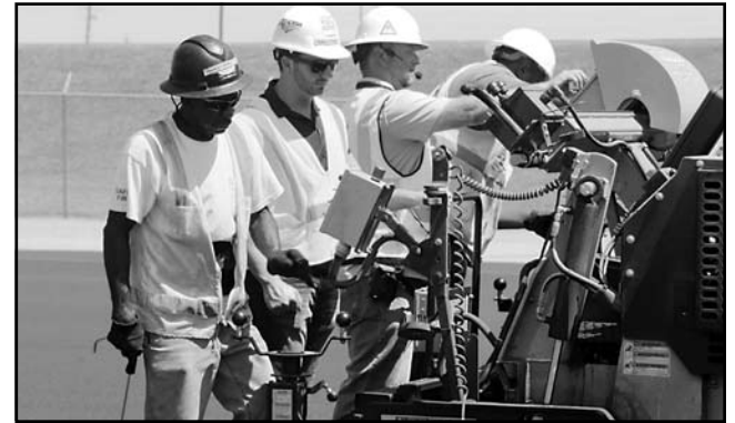
MATT 2ND IN (LAYING DOWN THE ASPHALT)
